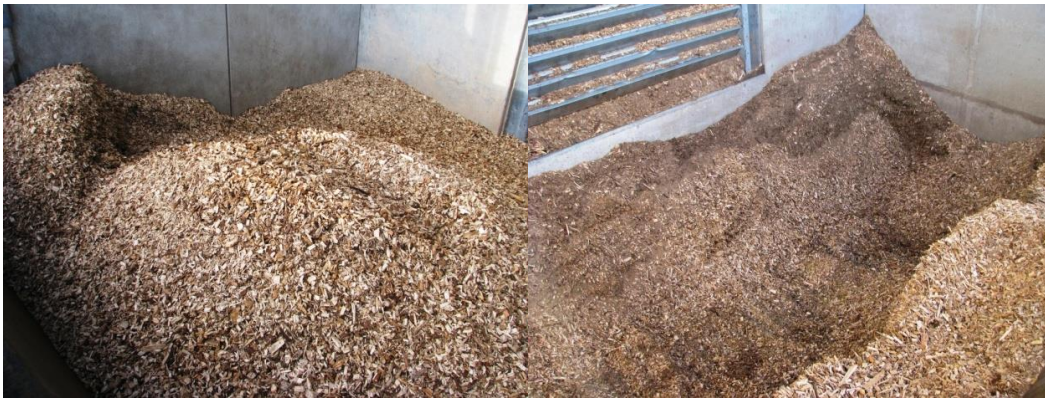
Figure 8.1-3: Wood chips in two of the four fuel intakes. (Photos: Morten Tony Hansen)
