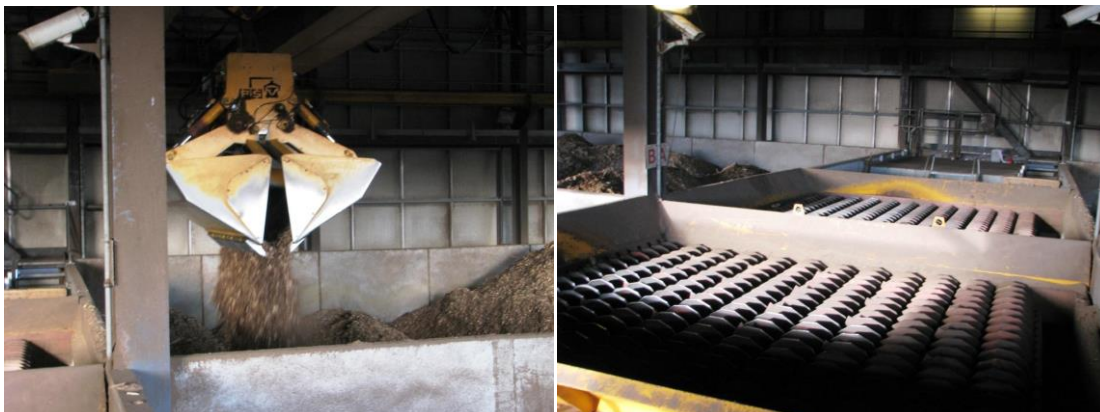
Figure 8.1-4: Automatic grab crane and rotating screens. (Photos: Morten Tony Hansen)
