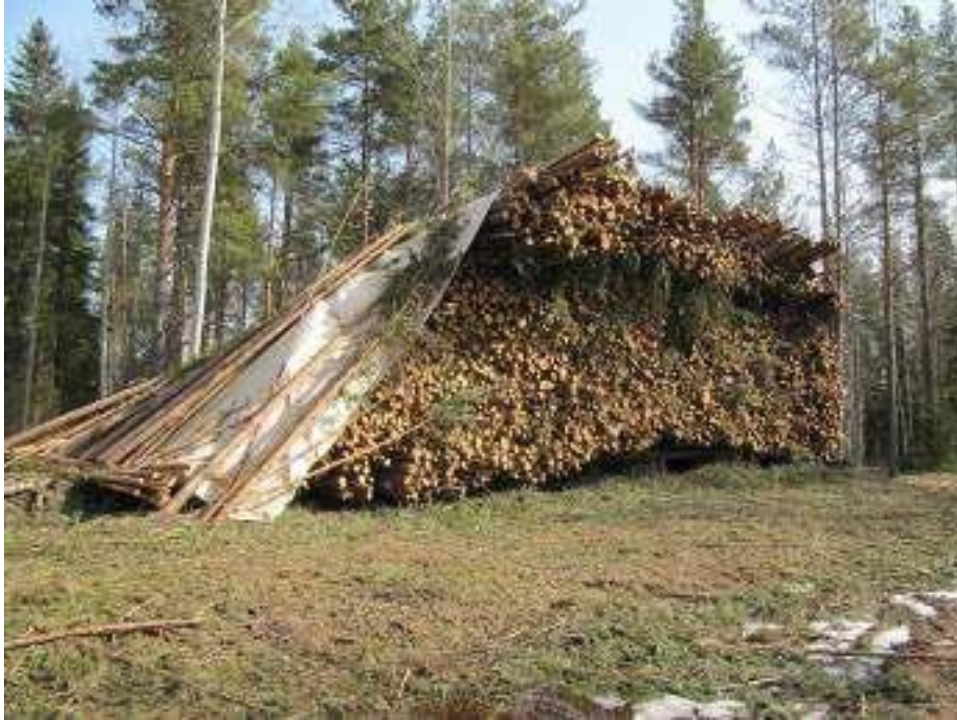
Figure 3. A proper wood fuel storage has 1) a cover made from kraftpaper; 2) base construction to create an airspace between the storage and the ground; 3) a peak to avoid rain pouring in from the front side, and 4) adequate height (4-5 metres). Source: AFO project ( www.afo.eu.com )
